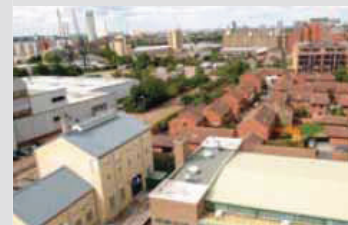
Barkantine Estate, London: retrofit community energy network using Combined Heat and Power (CHP) to service over 700 dwellings, a leisure centre/swimming pool and primary school.
