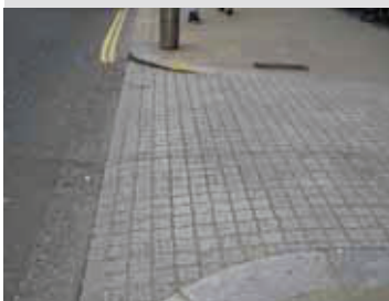
Below: raised crossing, High Street Kensington, London.
