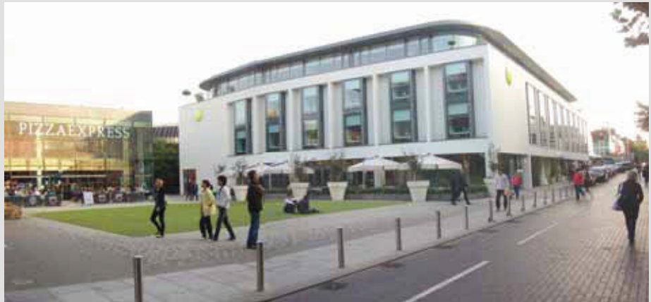
Jubilee Square, Brighton: overall design concept creates a coherent scheme with introduction of new activities and provision of new, flexible-use public space that attracts new users helps animate the public realm and increases natural surveillance.
