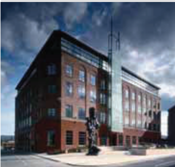
Central Sq, Newcastle: 1930's post office refurbishment.
